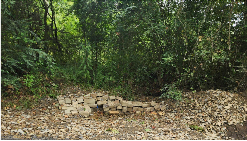
The spring at Walker's Station after repair by LeFlore County officials.
